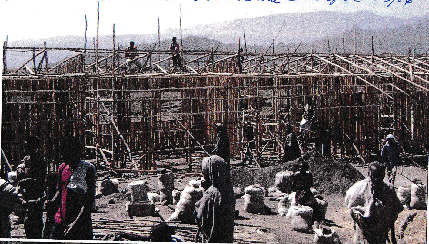
4 classroom block under construction Amhara Ethiopia 05/06
